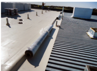
Class A Commercial Roof
