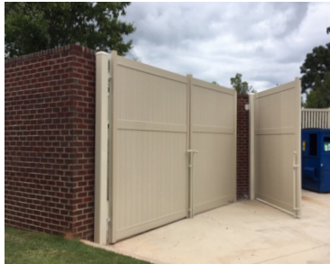
Enclosed garbage containment
